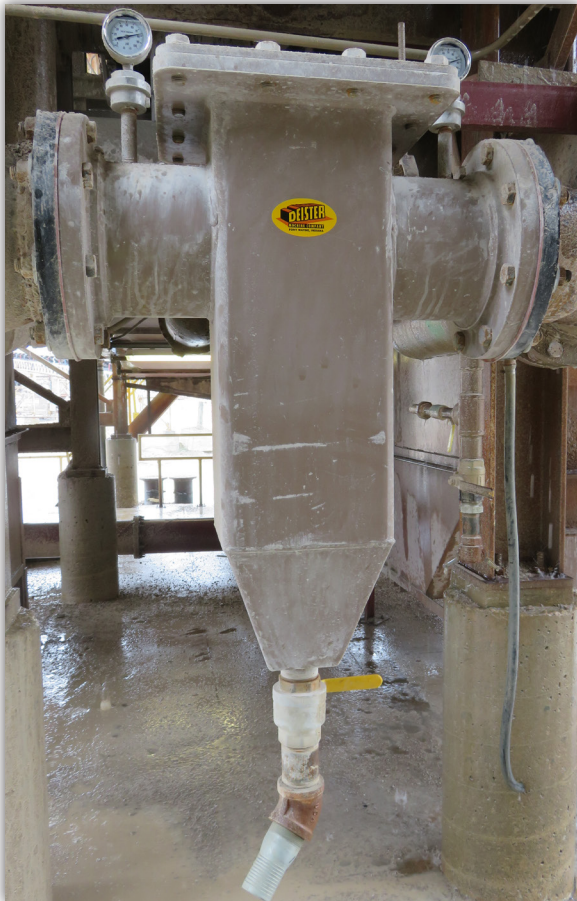
The Spray Water Strainer is installed at the base of the screen tower. Accumulated solids are purged through a cleanout valve, and strained water is supplied to the wash screens.
