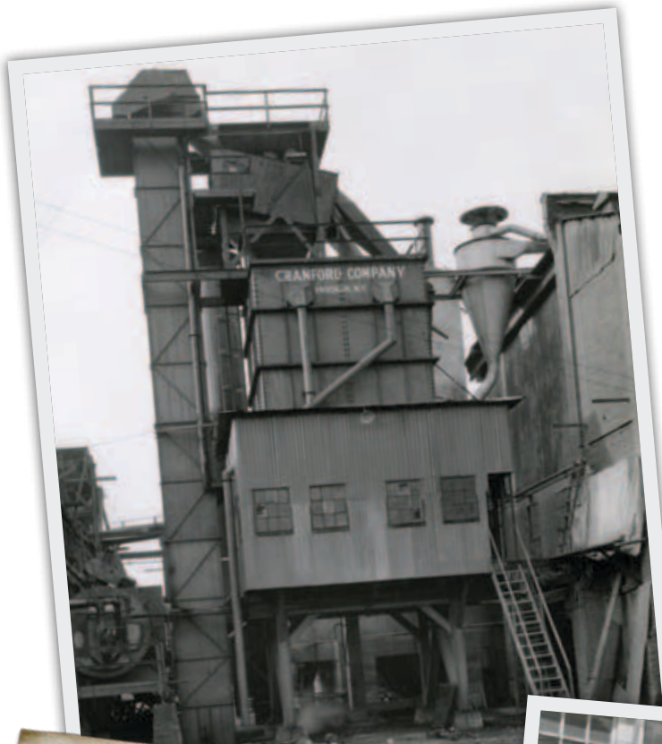
Circa 1933. An asphalt production site with a totally enclosed asphalt plant screen
